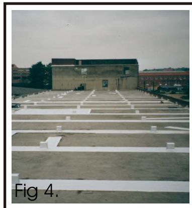
Fig 4. Here strips have been bonded over structural fault lines on this 1940's warehouse, saving the owners approximately £120,000 over the cost of a complete re-surfacing. We undertook this in 1993 and is still keeping the water out.
